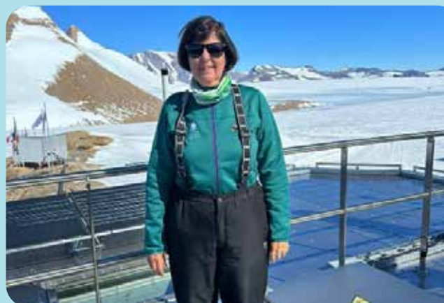
Above: The Minister inspects the solar installations on the roof of Princess Elisabeth in Antarctica.
