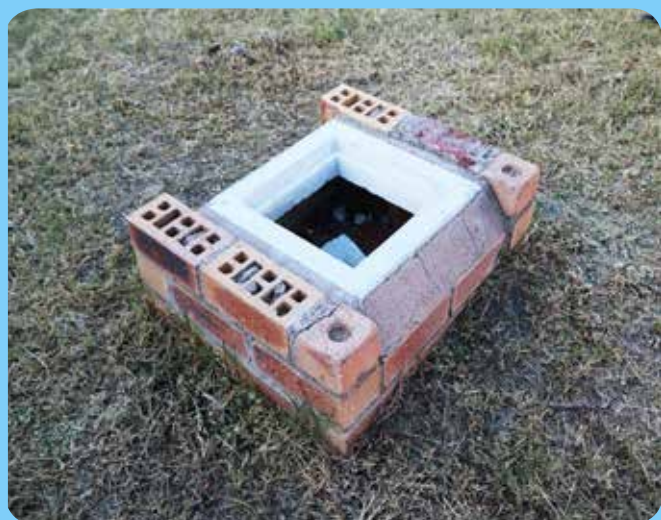
Above: The 130m deep bore hole that supplies water to the school garden and to the community when there is a water issue.
