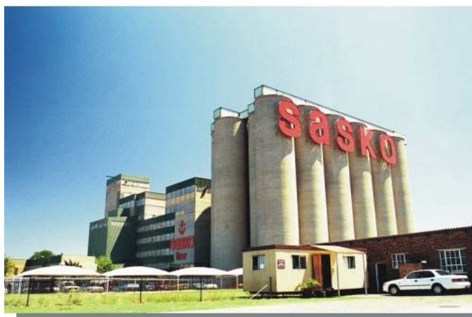
Chamdor Industrial Development
