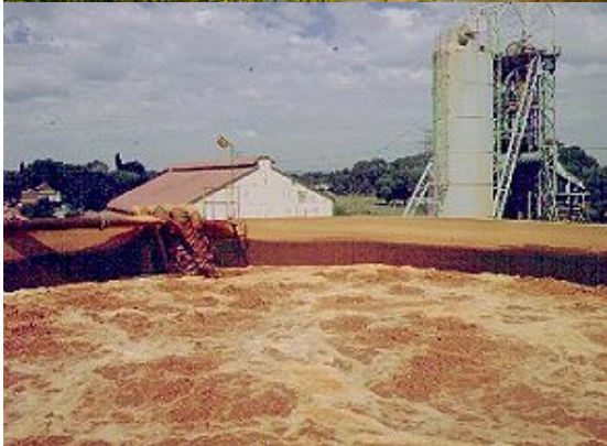
Current situation. Iron hydroxide-rich water is pumped from underground to a settling facility at the mine
