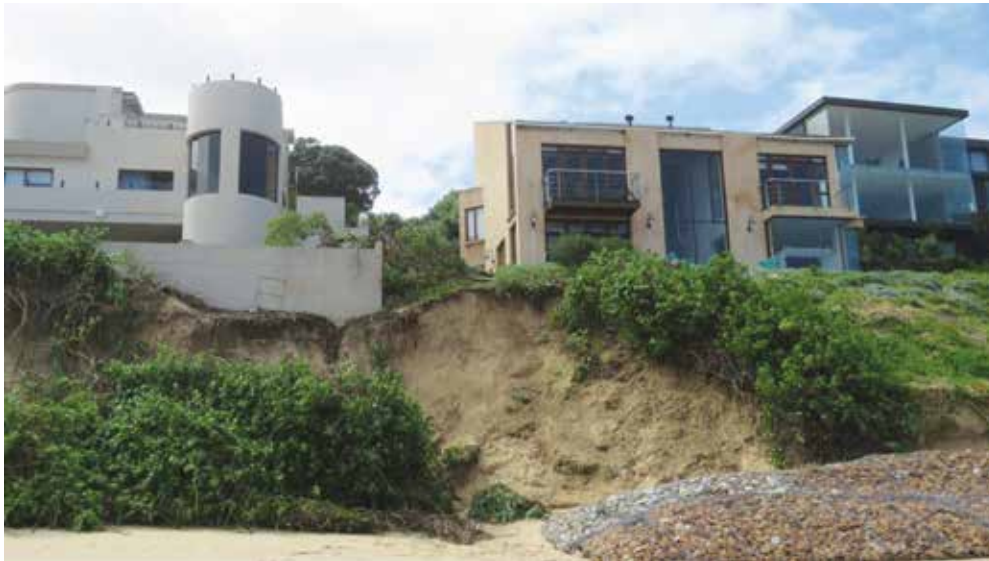
Figure 3: Example of sequential hazards
